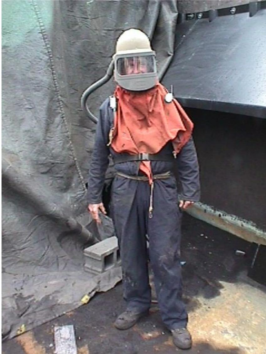
Figure 1. Blaster with personal protective equipment.
