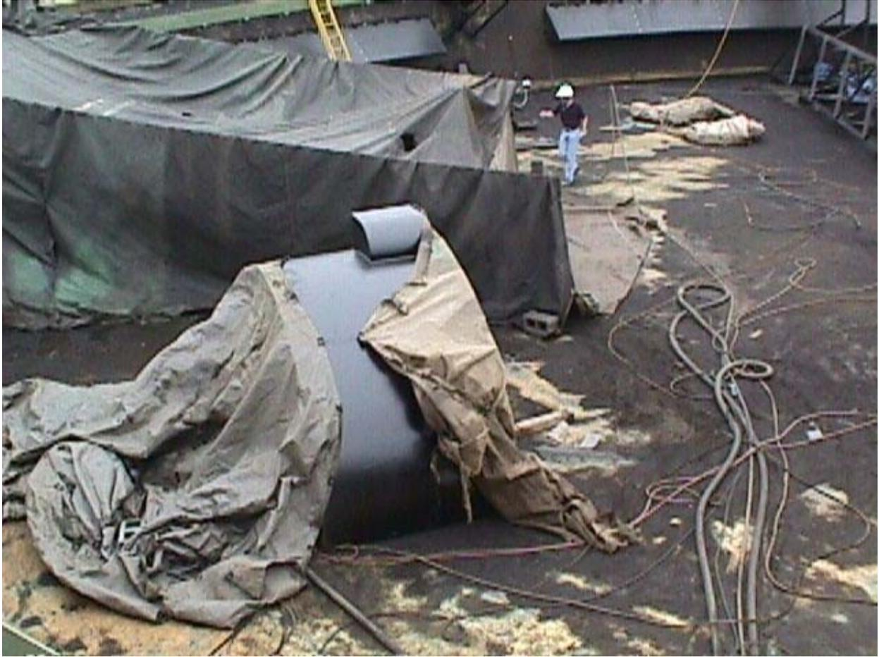
Figure 2. Containment tarps in place for abrasive blasting.
