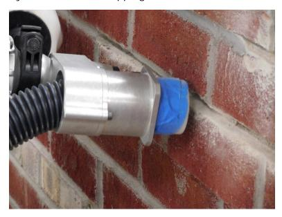
Figure 5 - Hood close to work surface
