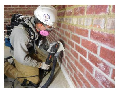
Figure 2 - Saw with modified hood (NIOSH photo)
