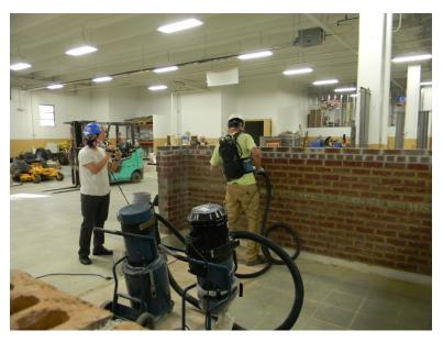
Figure 4 - Pre-separator (left) and vacuum cleaner (right) (NIOSH photo)
