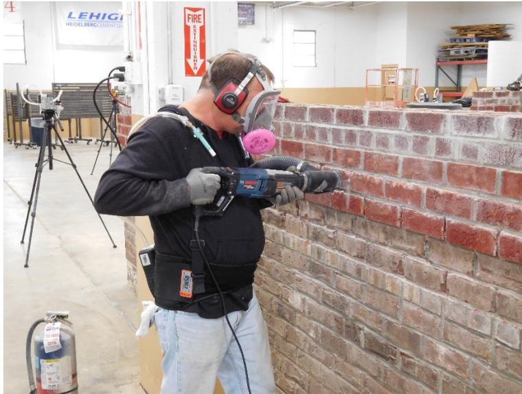
**Figure 2 - Hammer drill with shroud and bit (NIOSH photo)**
