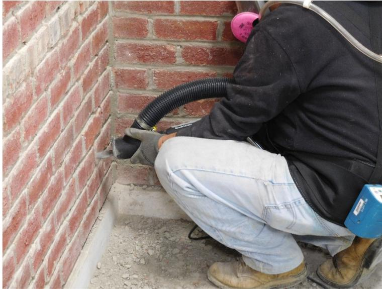
**Figure 4 – Removing mortar in an inside corner (NIOSH photo)**
