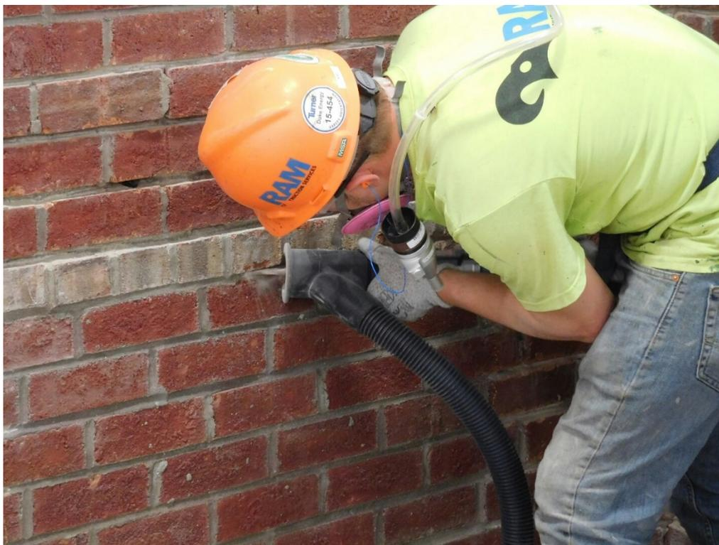
**Figure 5 – Cyclone sampler in the breathing zone (NIOSH photo)**
