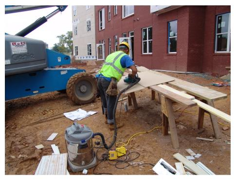
Figure 2 – A worker (cutter) cutting fiber-cement siding using a dust-collecting circular saw that was connected to a shop vacuum. Photo courtesy of NIOSH.
