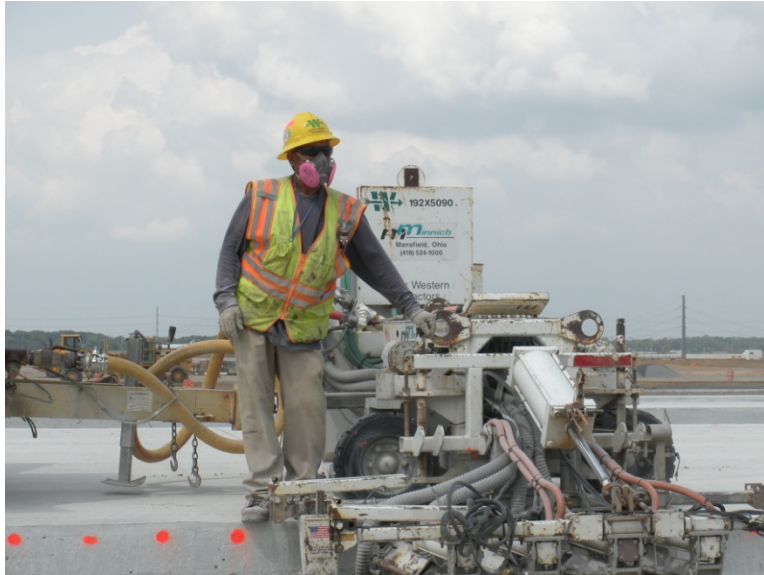
Figure 1 - Worker Operating Dowel Drill
