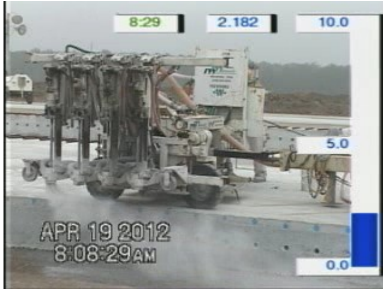
Figure 9 - Flushing Hoses and Hoods
