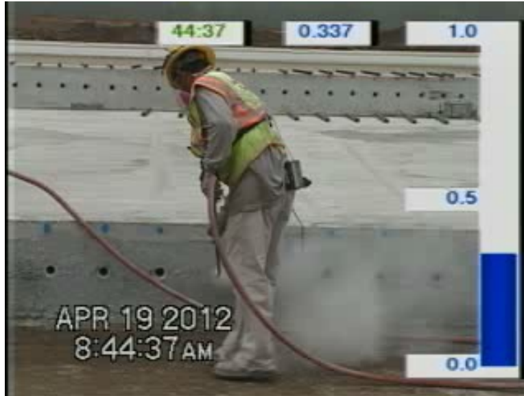
Figure 5 - Using Air Lance to Clean Holes
