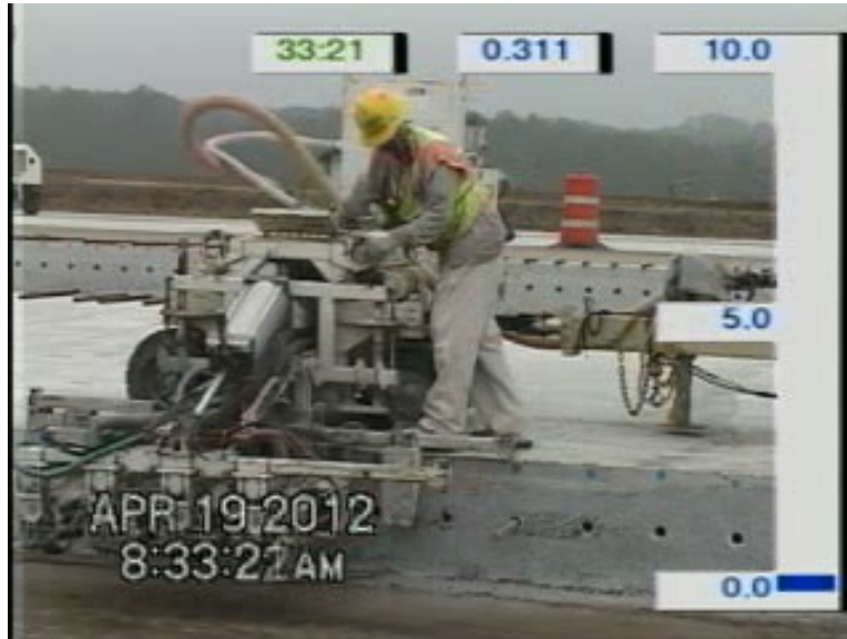
Figure 6 - Operating the Drill
