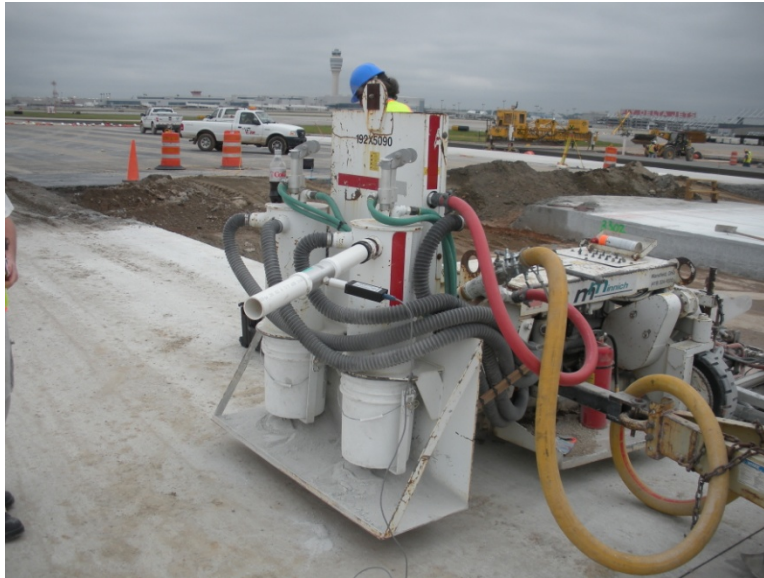
Figure 4 - Measuring Air Flow
