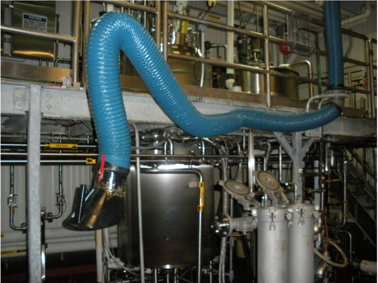
Figure 5. Hood located in the Laboratory mixing area
