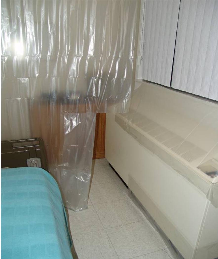
Figure 29. Photograph of the fan coil unit at St Joseph Memorial Hospital with expedient supply (shaded green) and exhaust (shaded red) tunnels installed.
