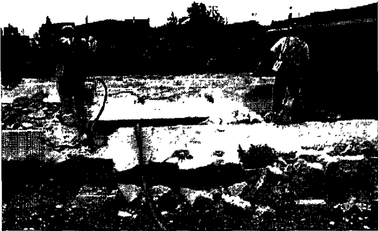
Figure 5 Workers during a wet trial
