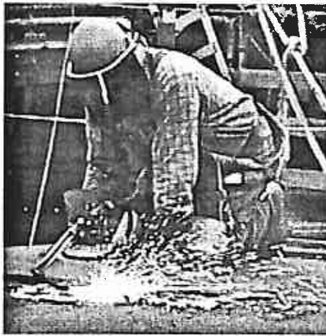
Figure 9. Torch cutting of steel deck
