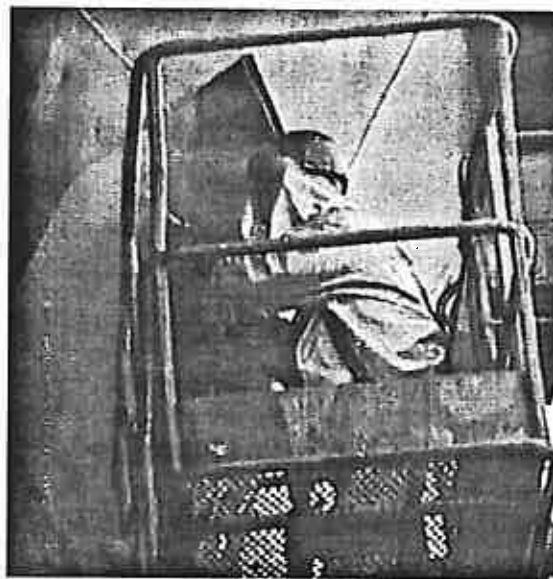
Figure 14. Worker using waterjet to remove paint from vessel
