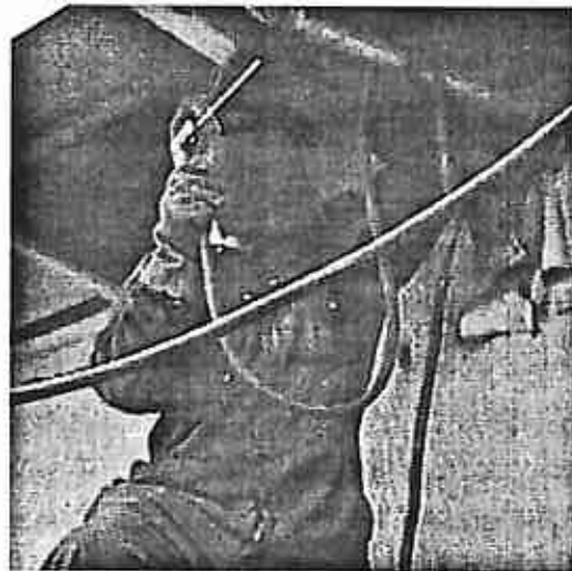
Figure 4. Pipefitter getting into position to weld
