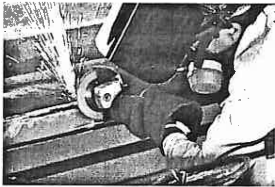
Figure 19. Grinding deck stiffeners for deck replacement
