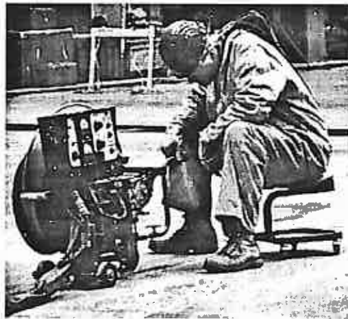
Figure 24. Worker running automatic welder while on stool
