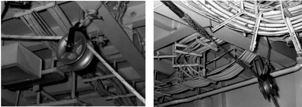
Figures 14a and 14b. Sheaves for Cable Pulling
