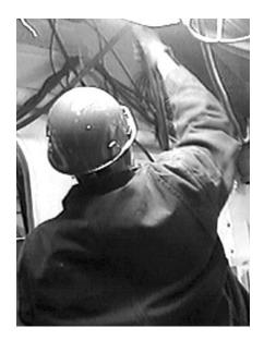
Figure 7. Cable Puller Standing, Feeding 3/4" Diameter Cable Over Head
