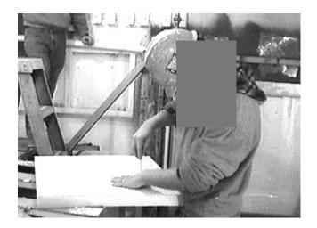
Figure 11. Insulator Cutter Using Knife to Cut Insulation
