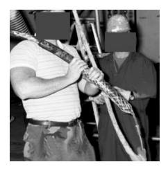
Figure 22. Cable Being Attached to Pull Rope
