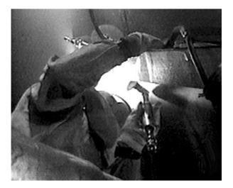
Figure 16. Tank Grinder Using 3 inch Offset Grinder
