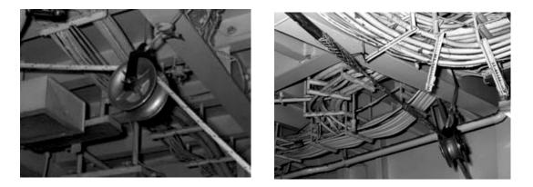
Figures 21a and 21b. Sheaves for Cable Pulling
