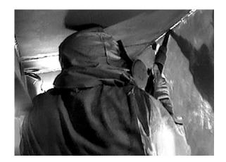
Figure 17. Tank Grinder Using Needle Gun Overhead
