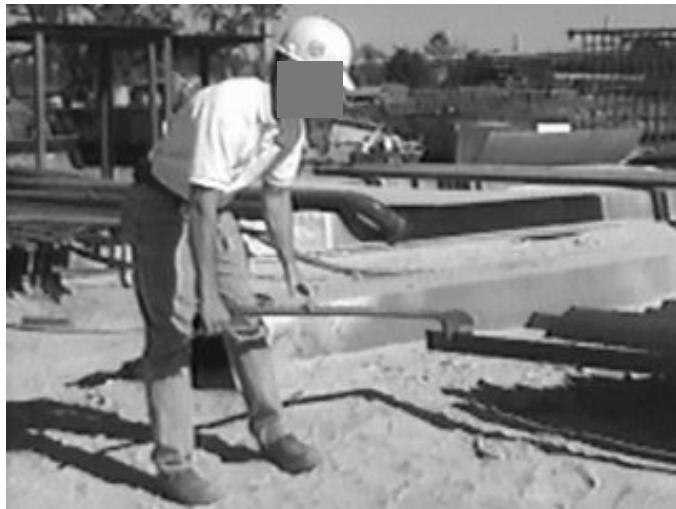
Figure 3. Gator Bar Worker Flipping Angle Iron from Side with Gator Bar
