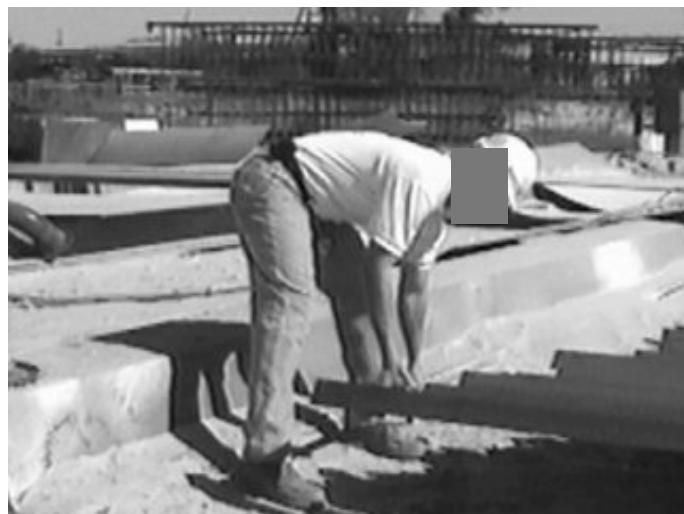
Figure 4. Gator Bar Worker Flipping Angle Iron from End with Hands
