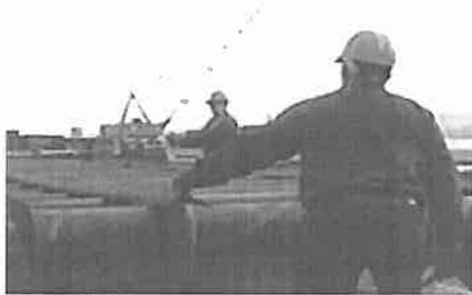
Figure 12. Workers positioning angle iron on roller conveyor
