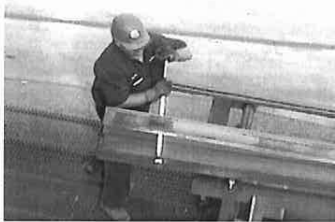
Figure 10. Separating angle irons with gator bar
