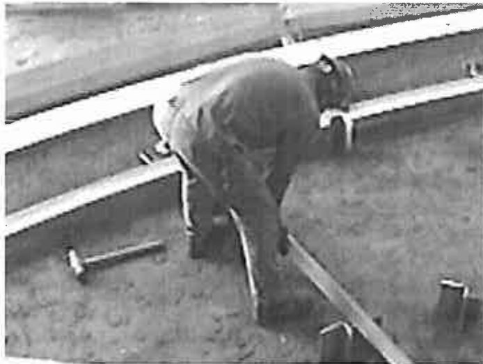
Figure 5. Worker placing smaller angle iron into jig
