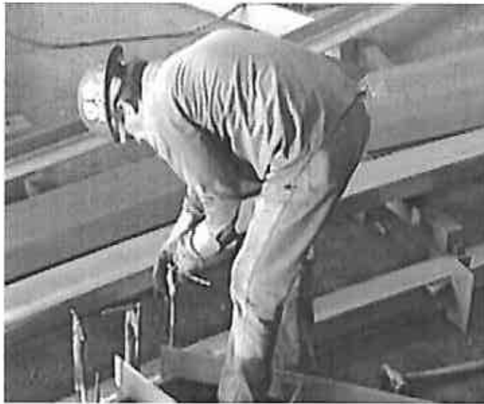
Figure 6. Shipfitter holding angle irons together with C-clamps
