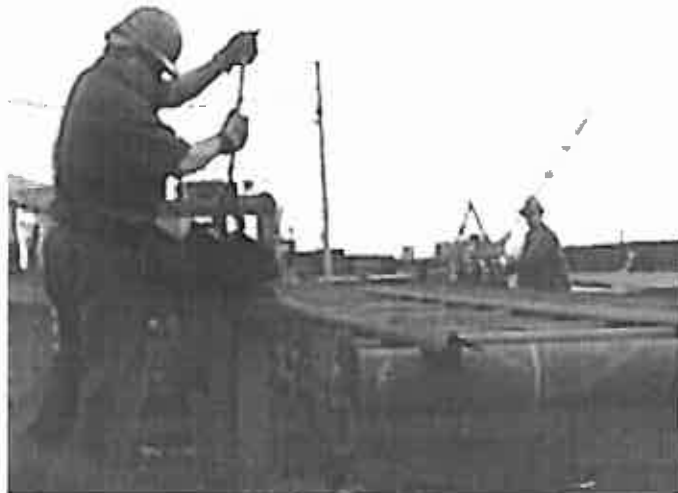
Figure 11. Flipping angle irons onto conveyor with gator bar
