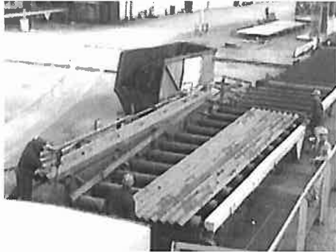
Figure 9. Steelyard conveyor system
