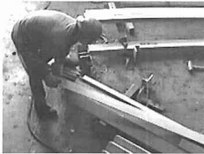
Figure 4. Worker moving angle iron from stockpile to jig
