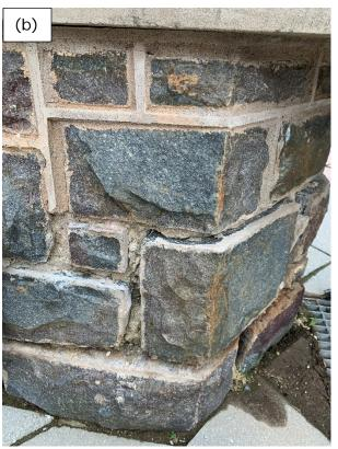
Figure 1 – (a) the stone wall building under renovation; (b) a closeup view of the wall where tuckpointing was to be conducted for the building renovation. Photos by NIOSH.
