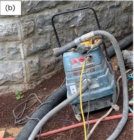
Figure 4 – (a) a handheld pneumatic wet grinder used to remove mortar; (b) a 13-gallon wet/dry vacuum cleaner providing LEV to a powered chisel. Photos by NIOSH.
