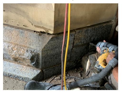
Figure 3 – A bricklayer using a powered chisel with LEV for tuckpointing. Photos by NIOSH.
