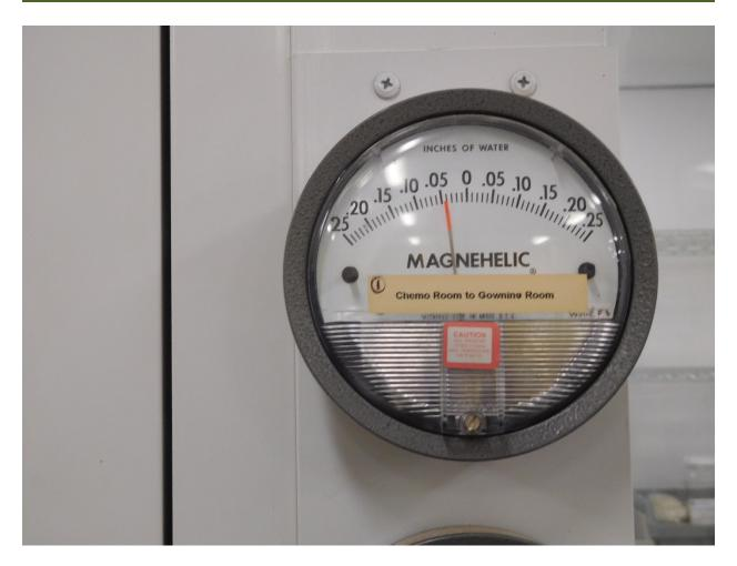
Figure 9. Magnehelic® pressure differential gauge read -0.04 inches of water for cleanroom (Photo credit: NIOSH)
