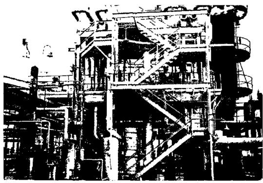
Figure 13. Production structure. Both reactors are visible (one left, one right side). Absorber in right background.
