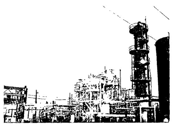
Figure 14. Production structure and absorber; one reactor is visible. Note exhaust gas return line on right side of absorber.
