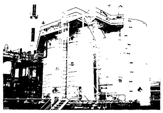
Figure 19. Formaldehyde storage tanks. Note dike and recirculation/loading pumps.
