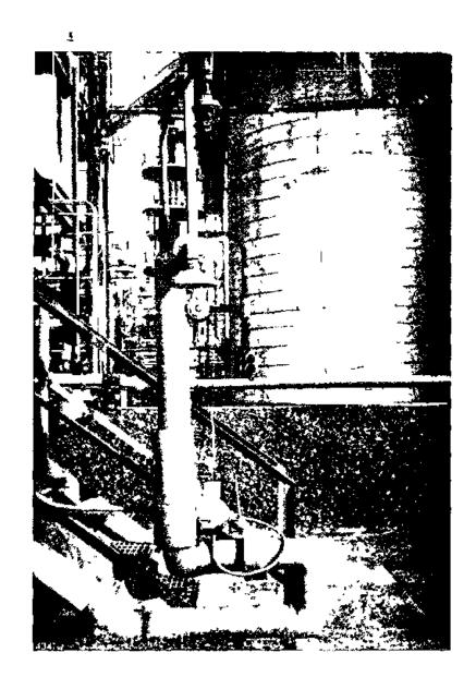
Figure 25. Eyewash and safety shower at truck loading area.
