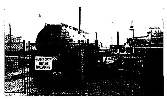
Figure 8. Methanol unloading area. Note gate and warning signs. Truck is in unloading process.
