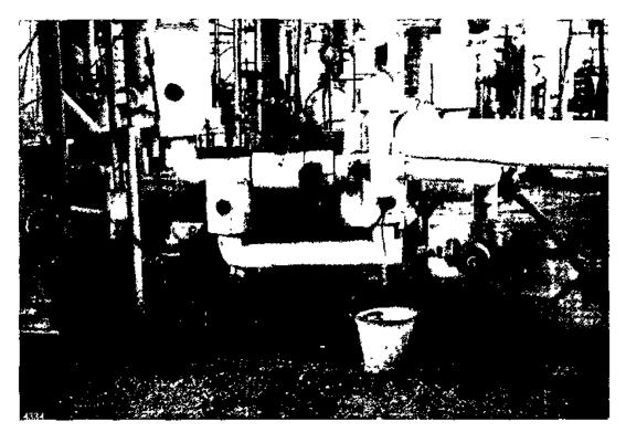
Figure 18. Absorber sample point. Note purge collection bucket and sample spout.
