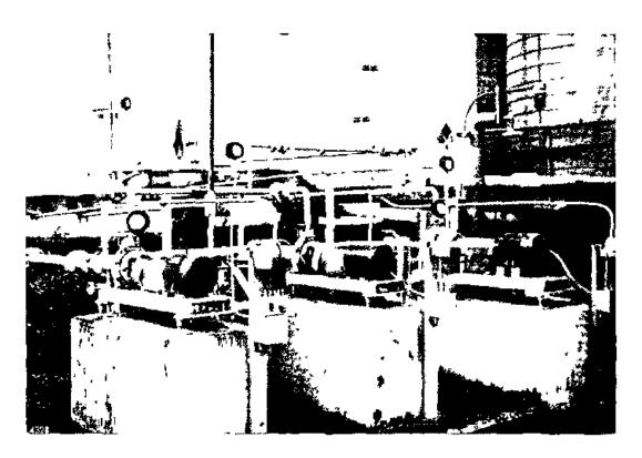
Figure 12. Methanol transfer (supply) pumps.
