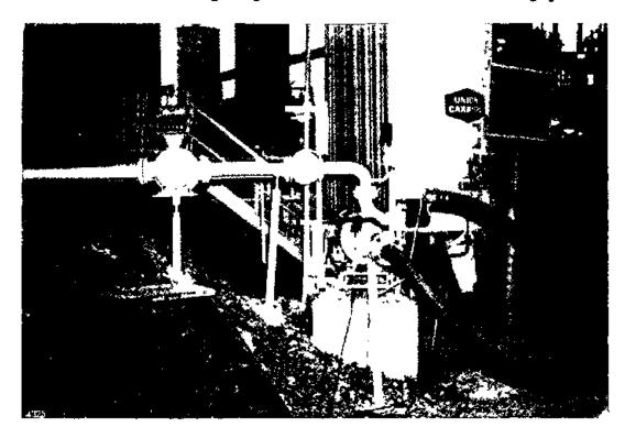
Figure 9. Reinforced rubber flexible hose used for unloading. Note quick-connect and grounding cable.
