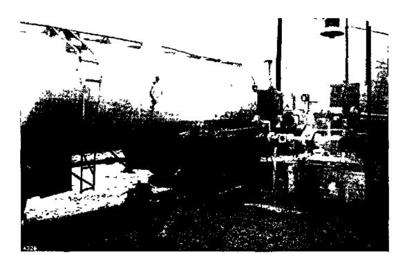
Figure 10. Tank truck connected by unloading hose to unloading pump.
