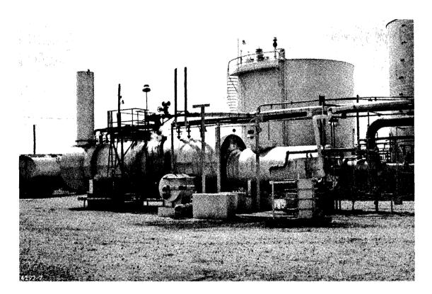
Figure 6. Incinerator for waste gas.
