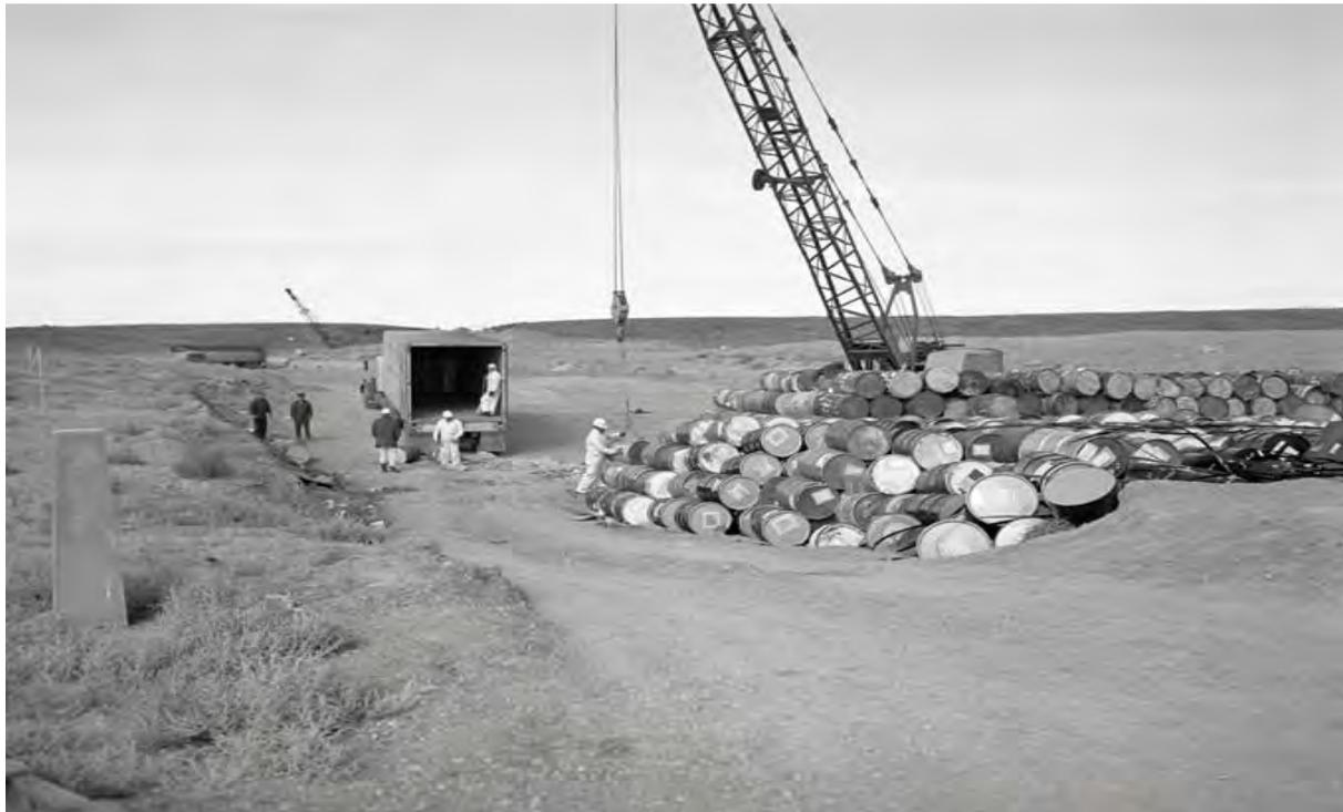
**Figure B-3. A Worker in Street Clothes Appears to Be Inspecting or Monitoring a 55-Gallon Drum of Rocky Flats TRU Waste (Burial Ground photo 1969b)**
