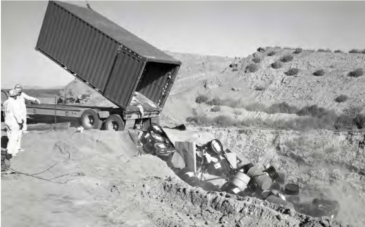
**Figure B-7. Trench Flooded with Spring Rain Runoff with Drums of Rocky Flats TRU Waste both Floating and Beached on the Side of the Pit (Burial Ground photo 1962)**
