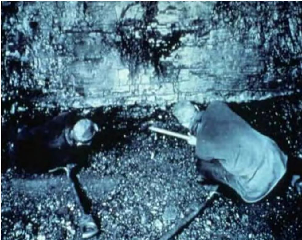
**Figure 25.** Undercutting coal with a hand pick in the early 20<sup>th</sup> century.
