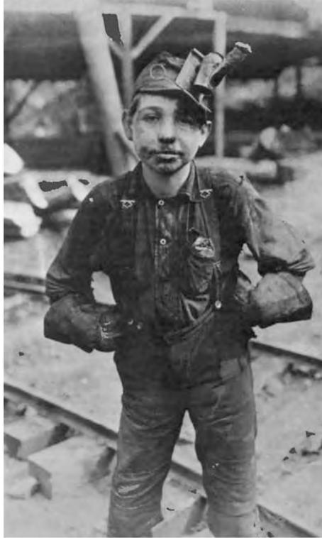
**Figure 2.** Child miner wearing cloth cap with open flame oil cap lamp, circa 1900.
