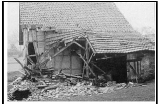
Figure 8. Damage to structure in Volkershausen directly above the shear zone (27).
