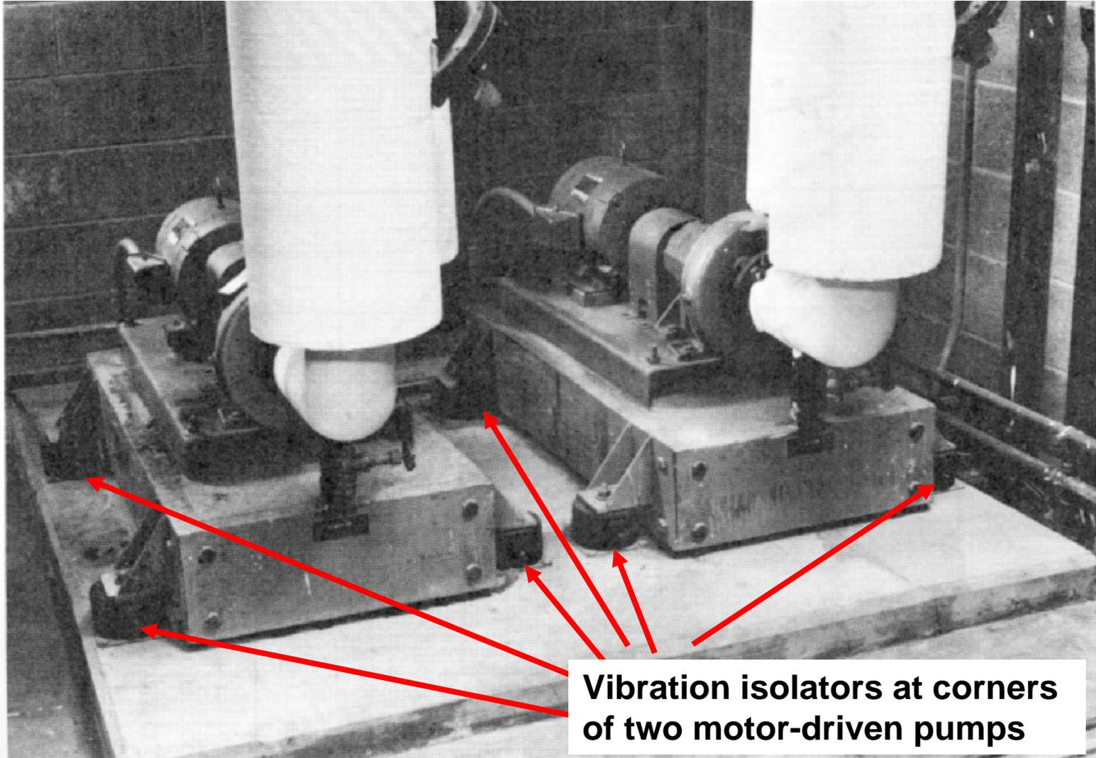
**Vibration isolators at corners of two motor-driven pumps**
