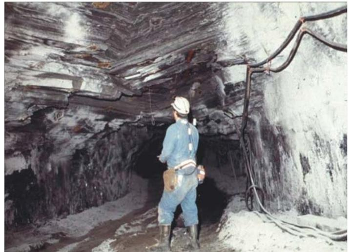
**Figure 1.—Severe cutter roof caused by horizontal stress.**
