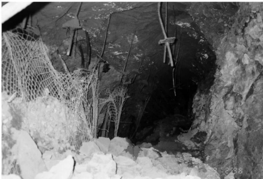
Figure 2. Rock burst damage in the 5750-05 stope. Note that both ribs, as well as the overhead sandfill, were damaged in this event.
