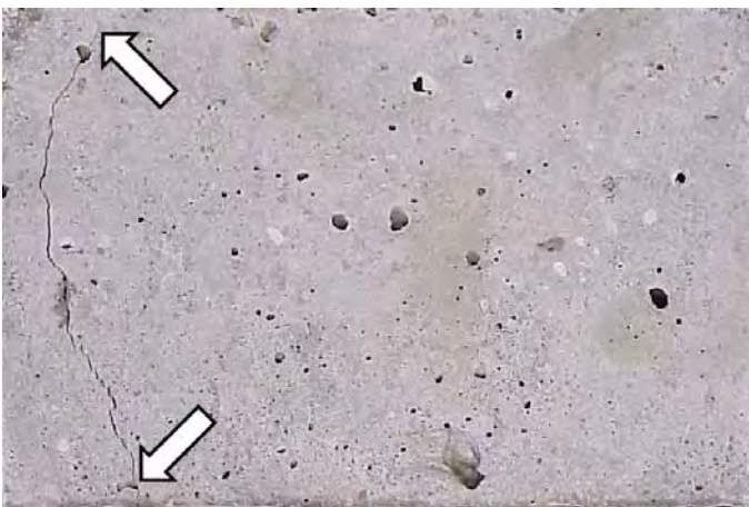
Figure 11. Shotcrete partial beam test specimen showing single side failure crack.
