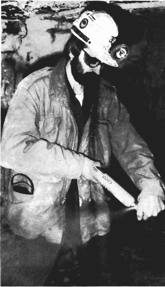
FIGURE 4. - Tracer gas being released from gas cylinder.
