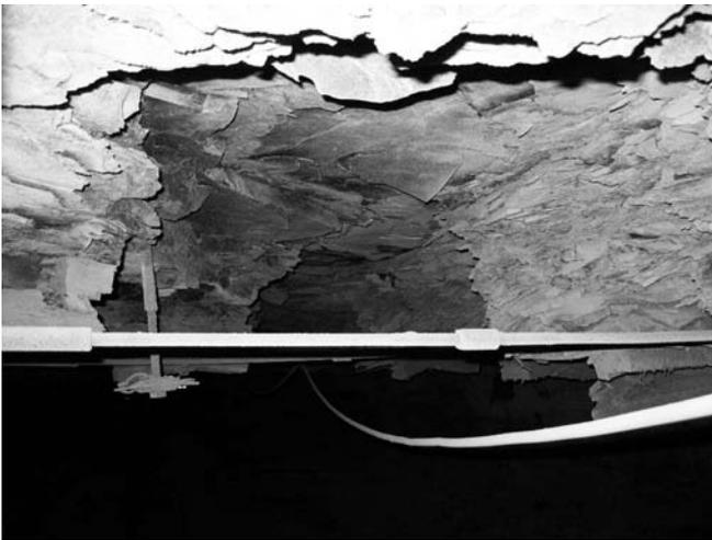
**Figure 7** — Gray shale weathers badly after protective black shale is removed.
