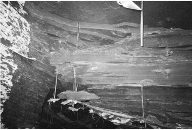
**Figure 6** — Roof fall in moisture sensitive roof.
