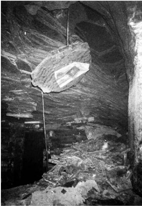
**Figure 9** — Severe guttering due to horizontal stress.
