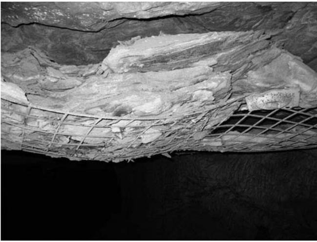
**Figure 12** — Roof screen loaded with rock.
