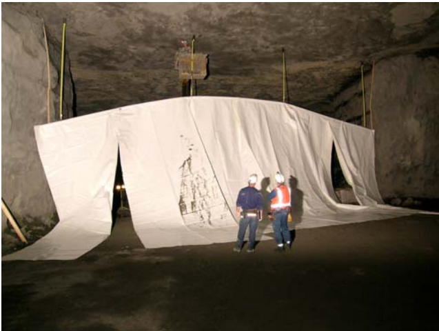
Figure 6. Raising the EZ-Up Curtain Stopping into position.
