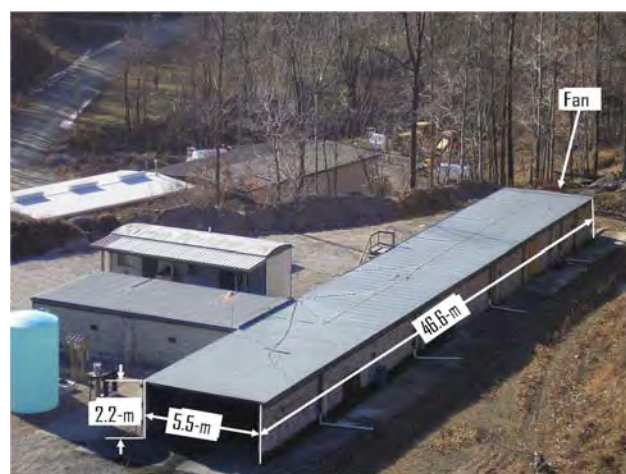
Figure 1. Exterior of Fire Suppression Facility
