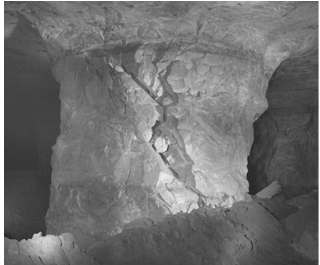
Figure 10 —Partially benched pillar that failed along two prominent discontinuities dipping at approximately 60^{\circ} .
