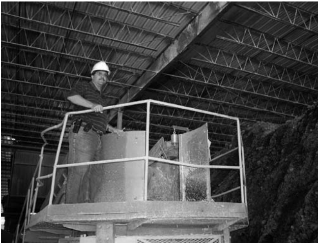
Figure 4a — Shredder tub with door installed.
