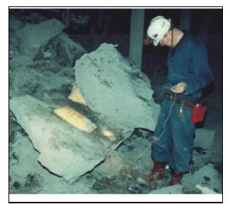
A Rock Buster is used to remove a roof fall.
