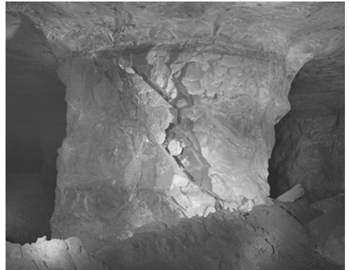
Figure 10. Partially benched pillar that failed along two prominent discontinuities dipping at approximately 60°.
