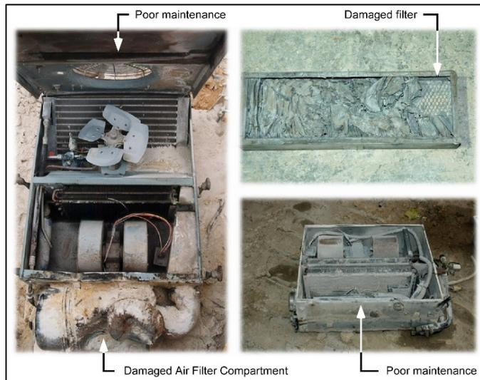
**Figure 1.** Examples of the poor quality and lack of maintenance on HVAC filtration and pressurization systems removed from mining machinery during various field research efforts. Photo in upper right corner shows the deterioration of a filter found in one of these units.
