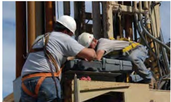
**Figure 2.** Installation of a uni-directional cab filtration and pressurization system. The uni-directional system delivers all of the filtered air into the enclosed cab at the roof and pulls all the recirculated air from the cab floor into the main filtering unit to be re-cleaned.
