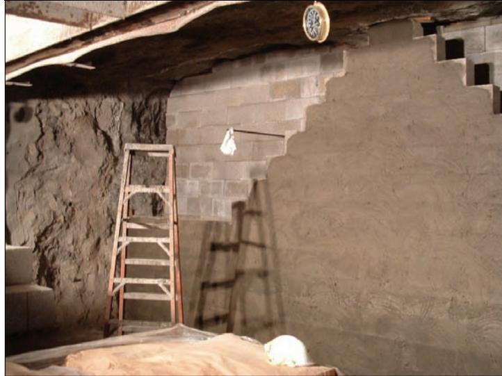
Figure 1.—The dry-stacked concrete block walls comprising the forms for the composite polyurethane seal.
