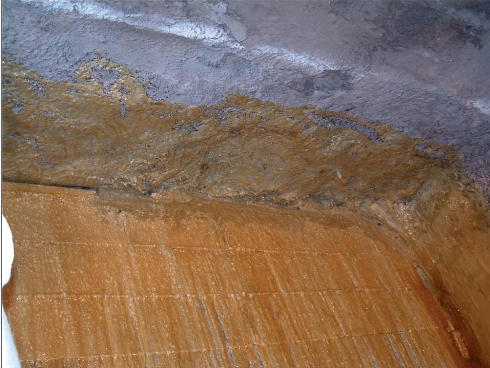
**Figure 3.—High-density (70 lb/ft<sup>3</sup>) polyurethane sprayed on roof, ribs, and back form wall.**
