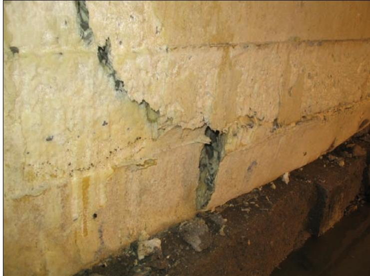
**Figure 15.—Fracture and damage observed along lower left side of polyurethane seal along top of bottom row of blocks.**
