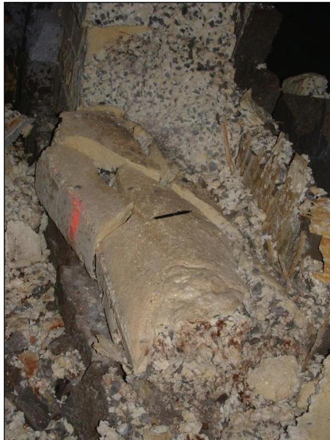
**Figure 16.—Internal damage along lower left side of polyurethane seal just above of the bottom row of blocks.**
