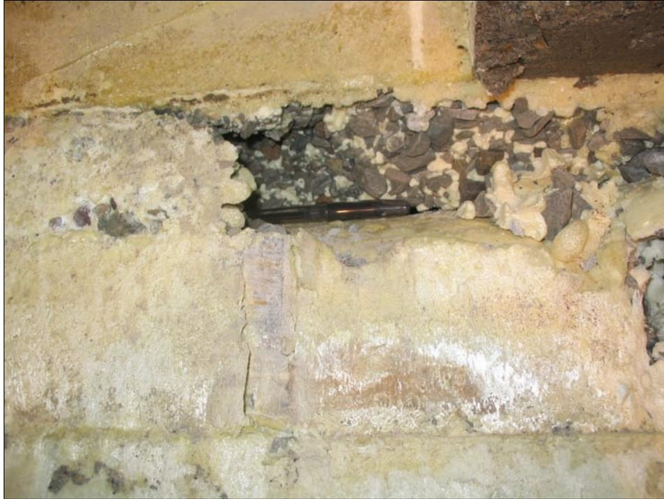
Figure 17.—High concentration of aggregate that is poorly bonded with polyurethane observed along upper right side of seal.
