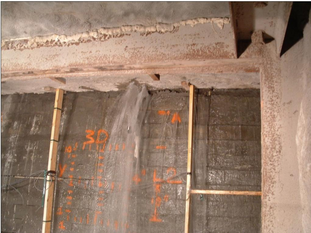
Figure 24.—Water leakage observed from failure zone along upper right side of the seal.
