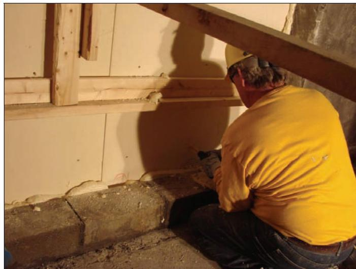
**Figure 25.—Injection of the two-component polyurethane foam at the perimeter and behind the rigid urethane board.**
