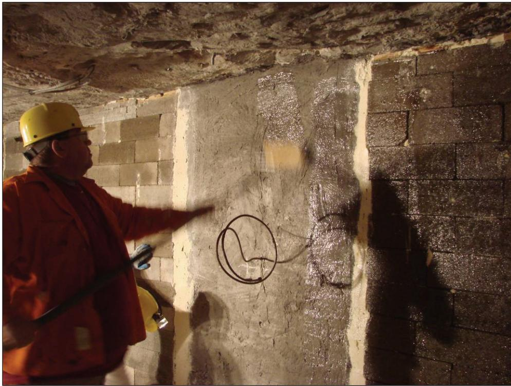
**Figure 27.—Applying the primer resin with a paint roller to the concrete block and pilaster.**
