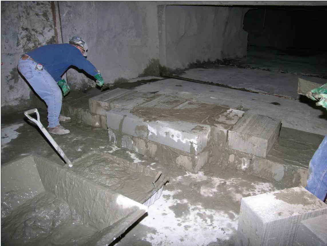
**Figure 13.—Full wet-bed construction on all horizontal and vertical block joints. The vertical block joints are staggered.**
