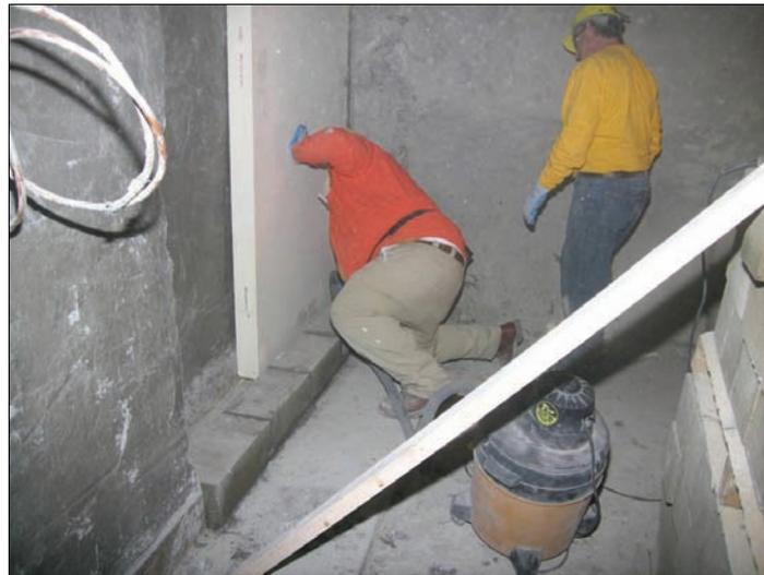
**Figure 24.—Positioning the rigid urethane board between the first course of concrete block and the seal.**
