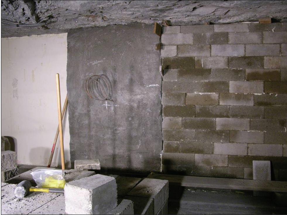
**Figure 26.—Completed block wall to the right of the pilaster and the installed rigid urethane board to the left.**
