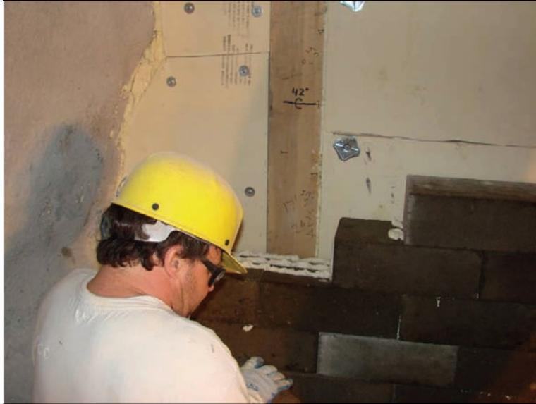
**Figure 19.—Construction of the solid-concrete-block wall. A one-component foam adhesive was used on all of the block joints.**
