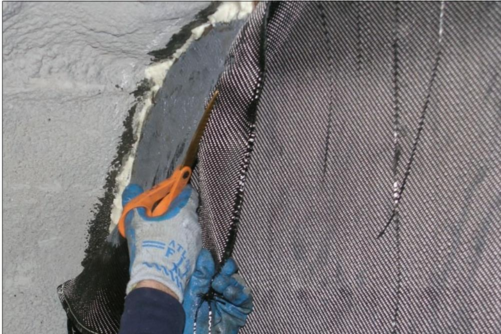
**Figure 22.—Cutting the woven CFRP base wrap to match the contour of the mine rib and roof.**
