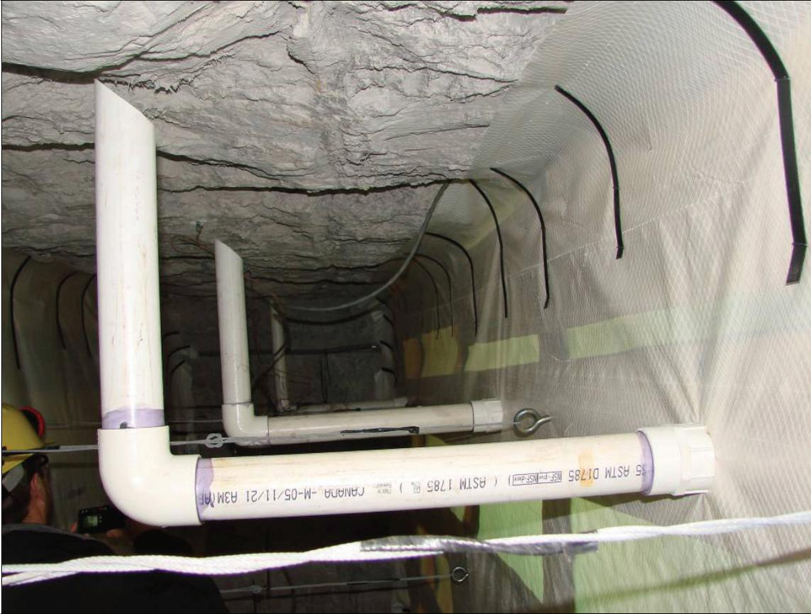
**Figure 7.—View between the two form walls showing the injection and bleeder pipes, the flexible metal straps holding the overlapped brattice tight to the strata, and the steel cable ties between the inby and outby form wall posts.**
