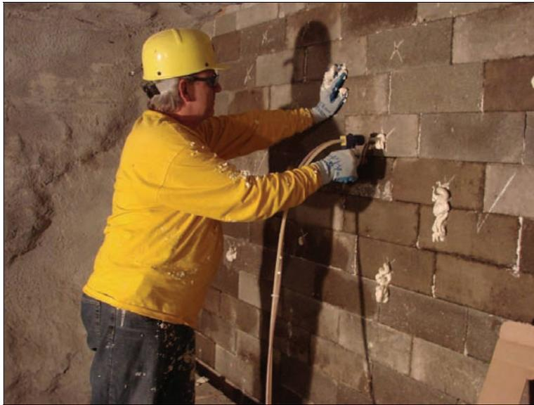
**Figure 20.—Injection of the two-component foam through the block to fill the 1-in gap between the seal and concrete block wall.**
