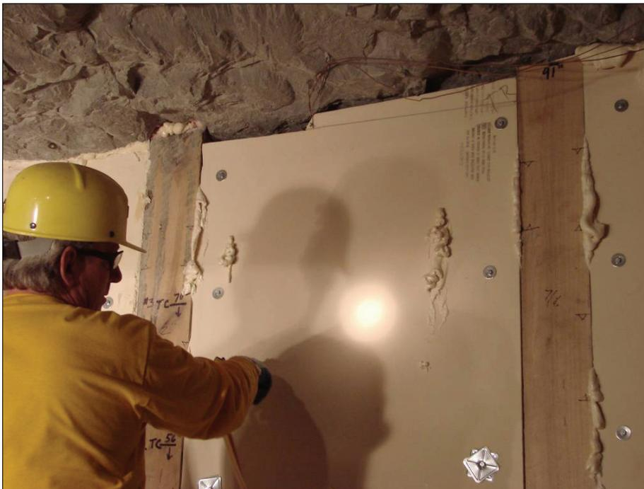
**Figure 18.—Injection of the two-component foam behind the rigid urethane board that was secured between the form wall posts with lag screws.**
