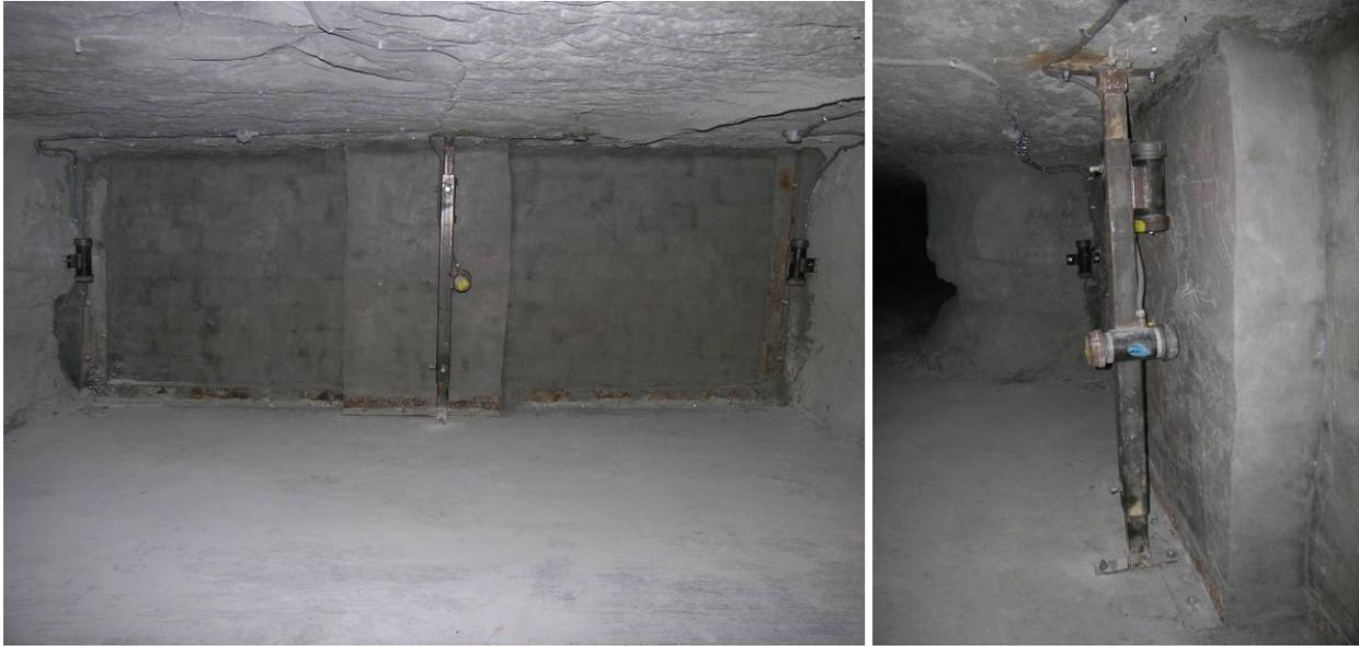
Figure 3.—Front view (*left*) and side view (*right*) of housings and mounts for the pressure transducers on the explosion (or C-drift) side of the low-density block seal in crosscut 3.
