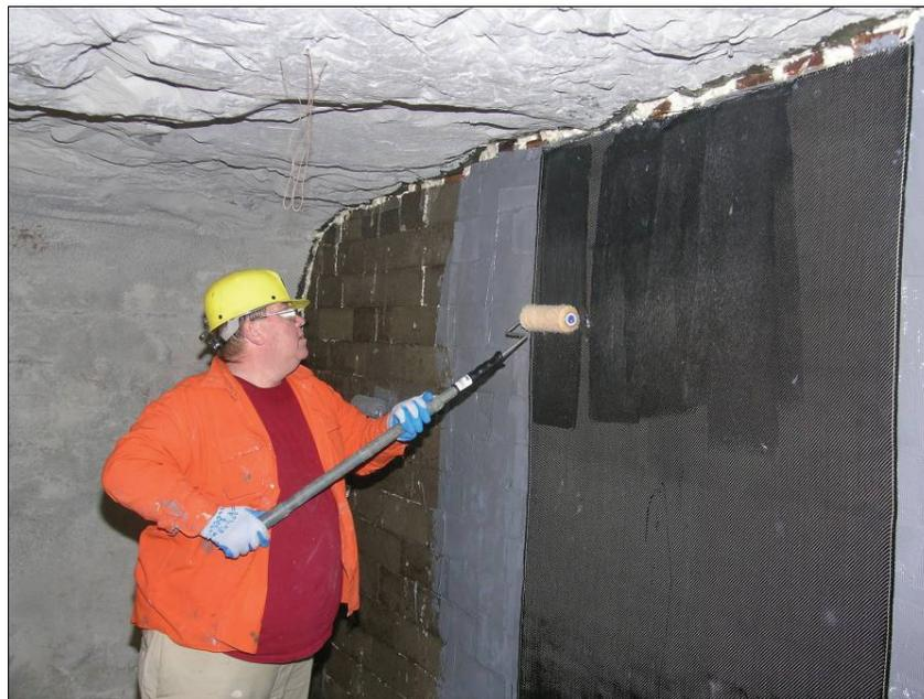
**Figure 21.—Applying the resin saturant coat over the CFRP base wrap. The light gray undercoating on the concrete block is the resin tack.**
