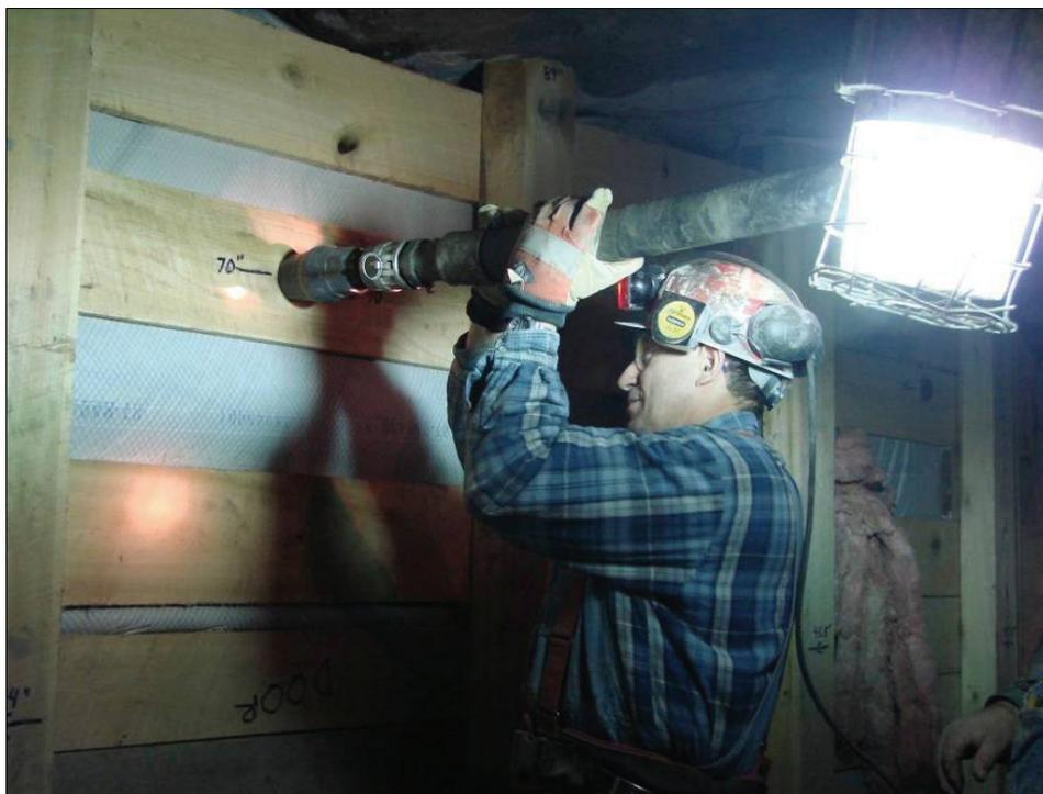
**Figure 11.—Connection of the slurry injection hose for filling the top third of the seal.**
