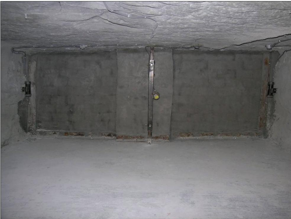
Figure 17.—Completed 24-in-thick, low-density block seal as seen from the C-drift (explosion) side.
