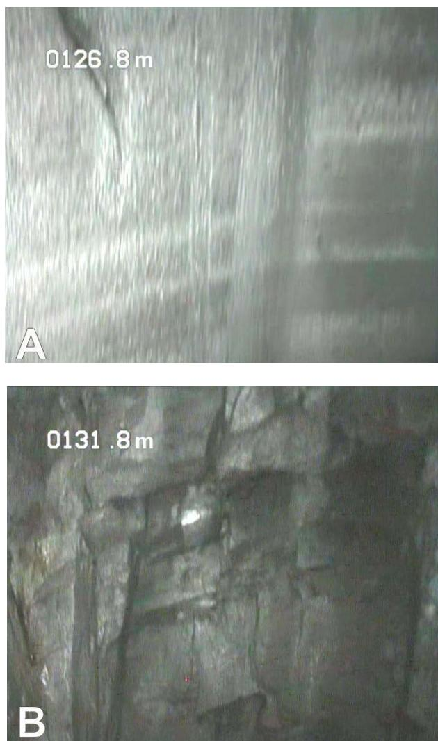
Figure 5.—No overbreak (A) versus overbreak (B) in a raise-bored shaft.
