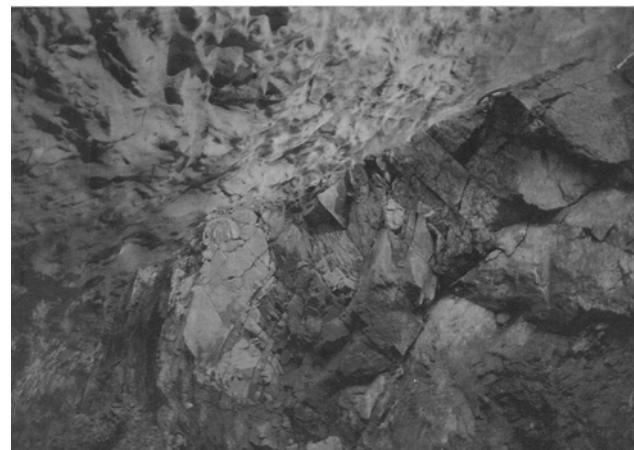
**Figure 6.—Example of a well-jointed rock mass with most typically  $J_n = 9$  (three sets of joints) and  $J_r = 2$ , seen in the Gjøvik Olympic cavern of 62-m span. Note the deep overbreak in the 25-m-high arch and the use of B + S(fr) permanent support [Barton et al. 1994].**
