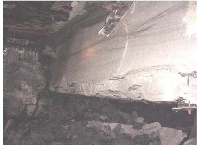
**Figure 8.—Damage caused when open entries were subsided.**
