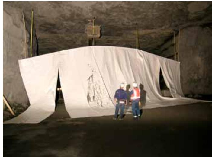
Figure 2.—Raising the EZ-Up curtain stopping into position.
