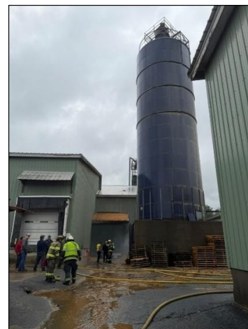
View of operations from recent silo incident. Photo by the fire department.
