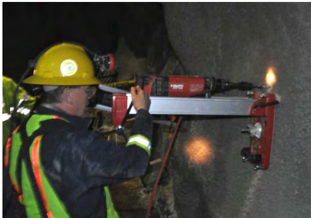
Figure 63. Dry drilling the installation hole for the epoxied stud pull anchor.
