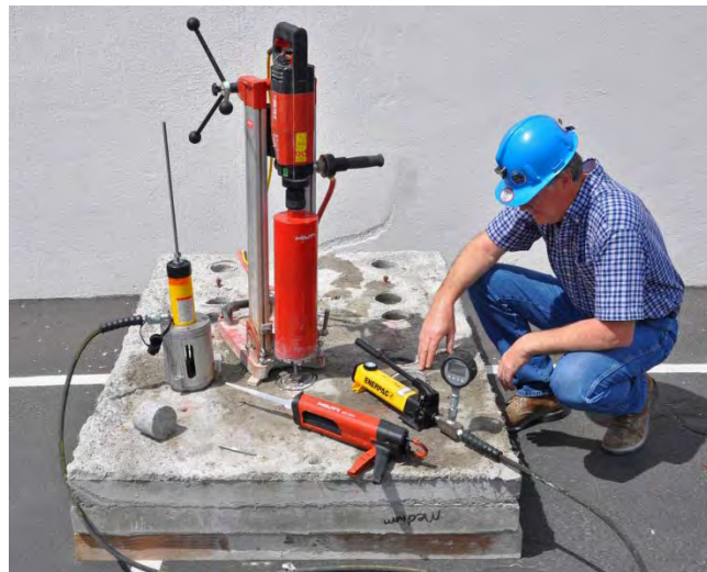
Figure 53. Operation of overcoring and direct-tension test equipment.
