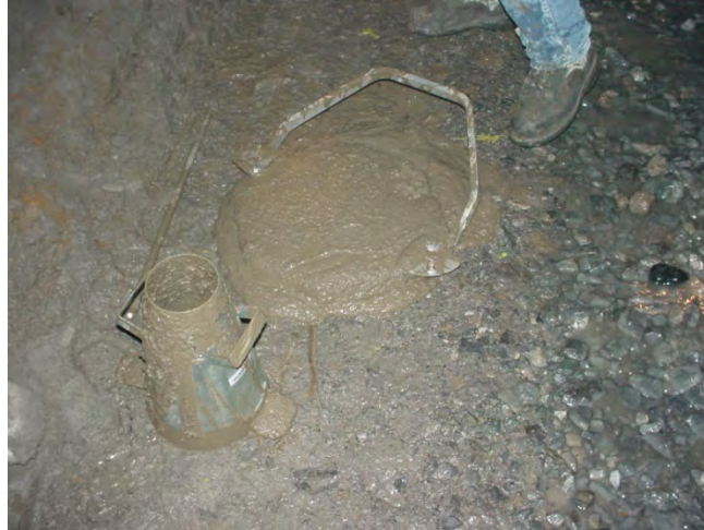
Figure 33. Slump test with wet mix shotcrete showing a 292-mm (11.5-in) slump; typical slump is 100 to 200 mm (4 to 8 in).
