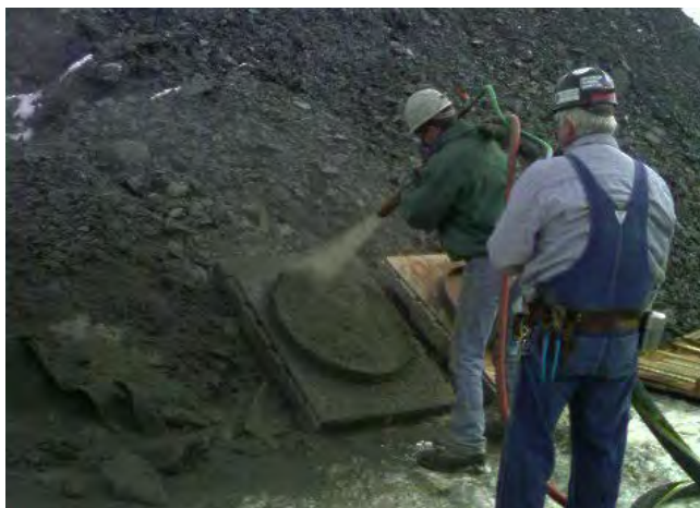
Figure 87. Spraying round panel forms with a dry mix shotcrete.
