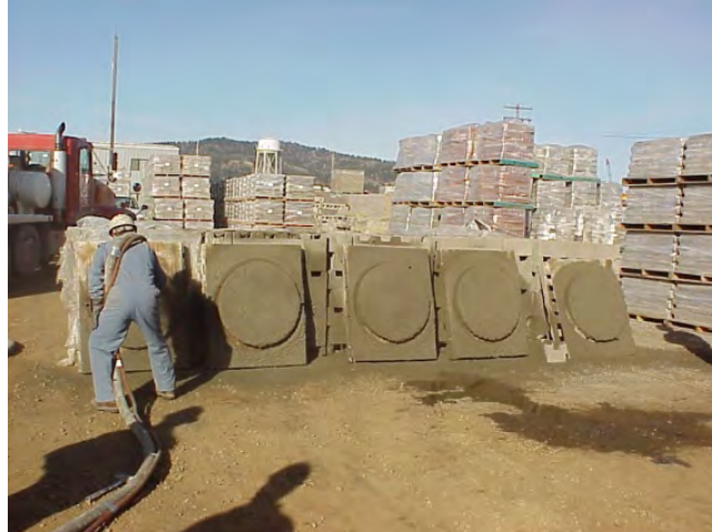
Figure 91. Spraying round panel forms with wet mix shotcrete.
