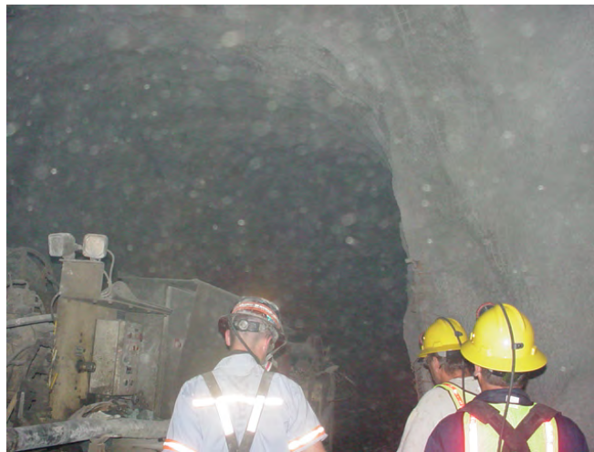
Figure 4. Final in-cycle application of wet mix shotcrete.
