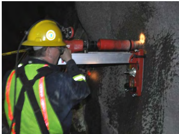
Figure 55. Wet drilling with diamond core bit.
