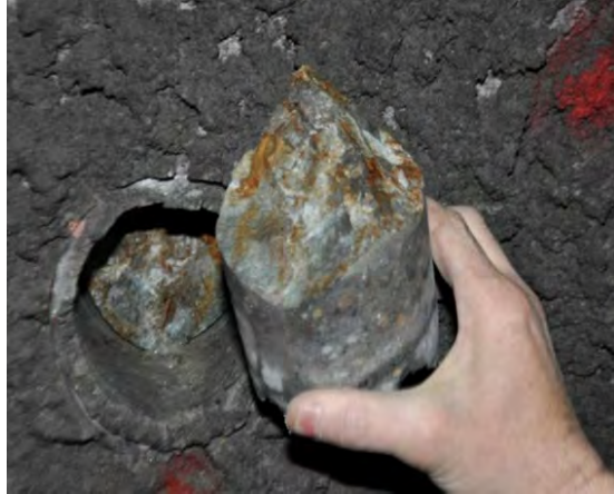
Figure 69. Adhesion test #3: drill hole and core indicating a tensile failure located primarily in the host rock.
