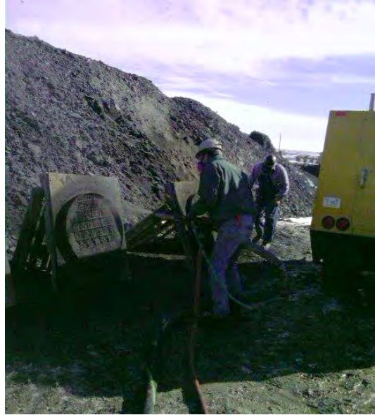
Figure 96. Shooting wet mix shotcrete into a round panel form with wire mesh reinforcement.
