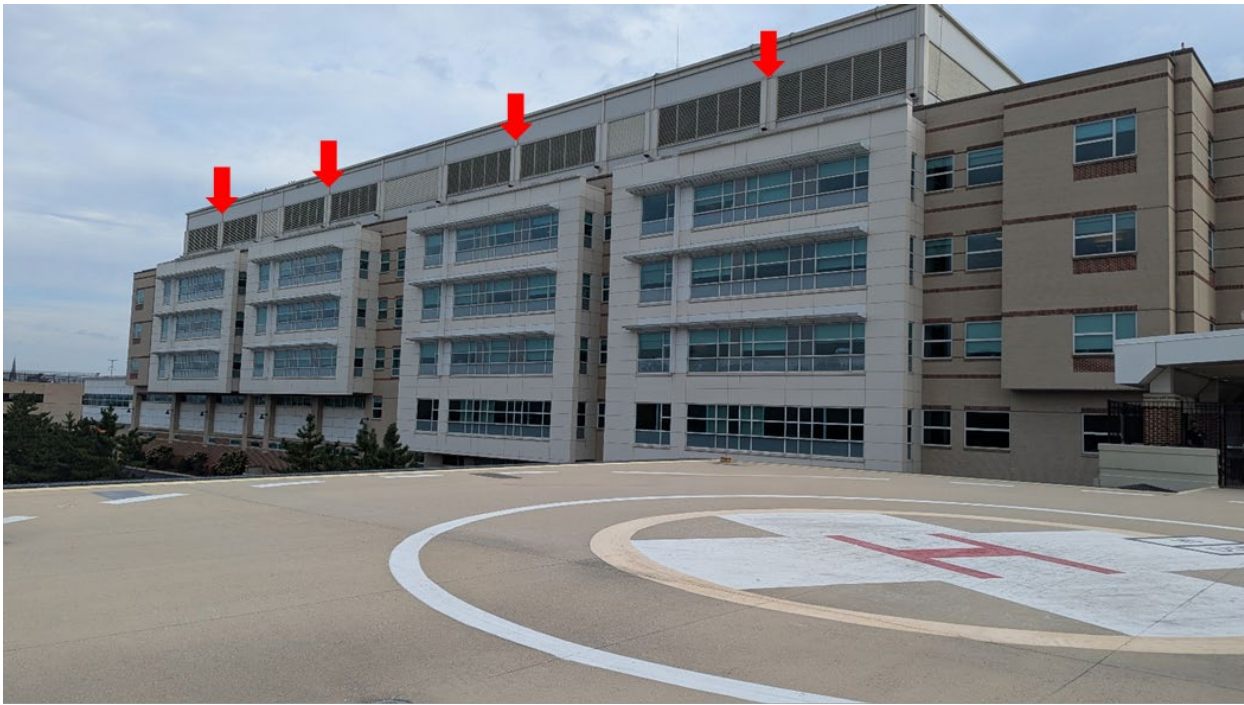
Figure 1. Photo taken from helipad showing the location of four pairs of rectangular outdoor air intake grilles (red arrows) located at the penthouse level on the southwest side of the building. (This photo was altered to remove the name of the hospital on the helipad.) Photo by NIOSH.
