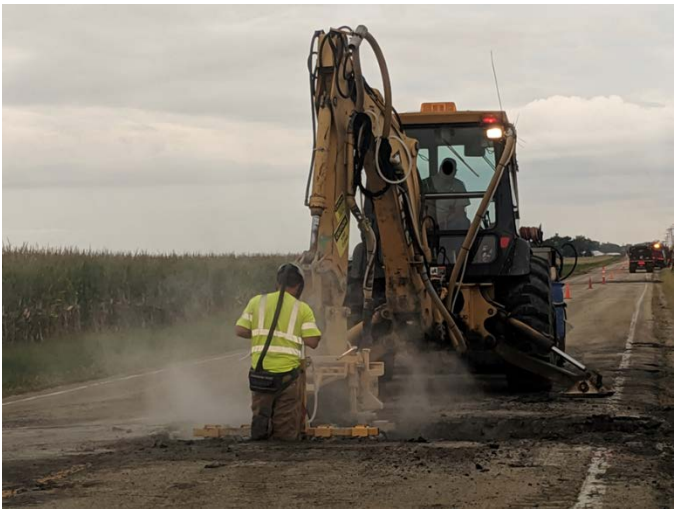
Figure A2. Employee operating the drill rig. Photo by NIOSH.
