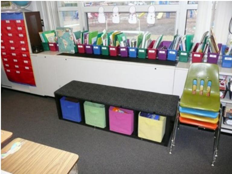
Figure A9. Storage cabinet (on floor) and teaching supplies (on top) blocking air intakes on a classroom unit ventilator. Photo by NIOSH.
