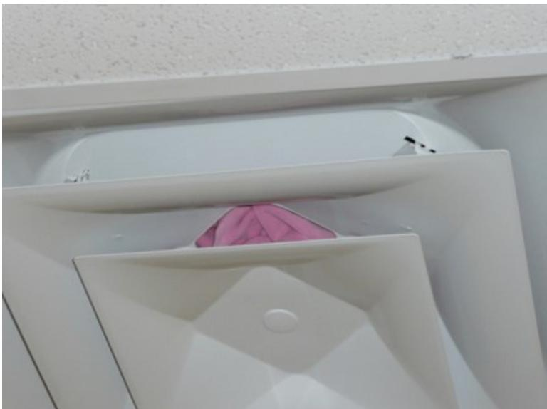
Figure A10. A blocked ceiling mounted diffuser in an office. Photo by NIOSH.
