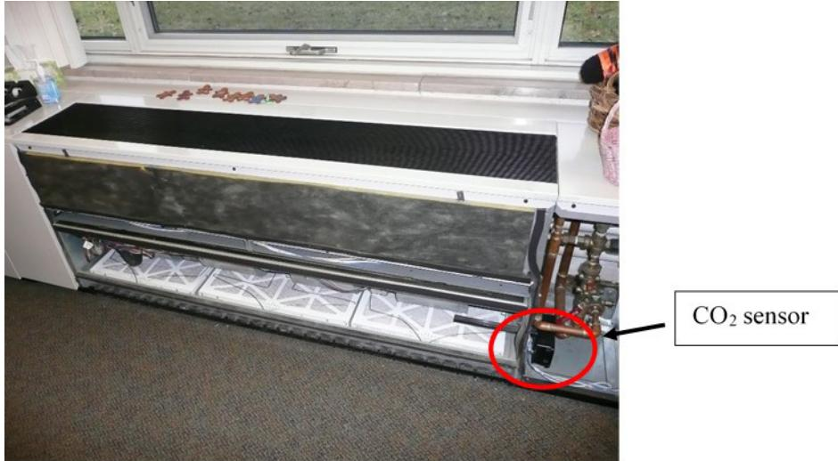
Figure A8. Interior of a typical classroom unit ventilator. Photo by NIOSH.
