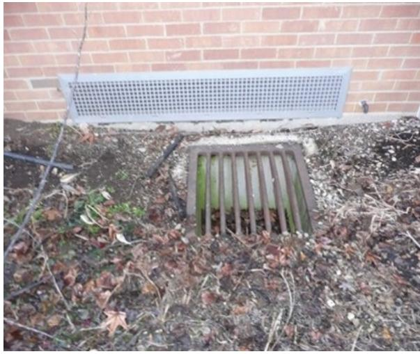
Figure A7. Debris in shallow dry well near outdoor air intake for classroom. Photo by NIOSH.
