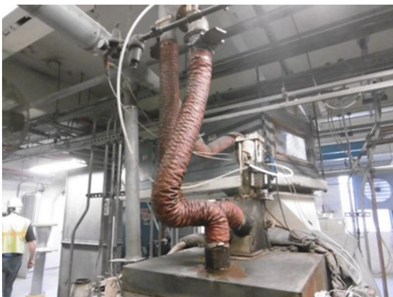
Figure 3. Excess flexible duct and bends in duct above mixer #2. Photo by NIOSH.
