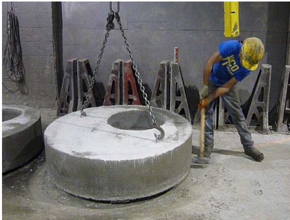
Figure 3. Drycast operator using a sledgehammer to loosen and release the base plate from the dried form. Photo by NIOSH.
