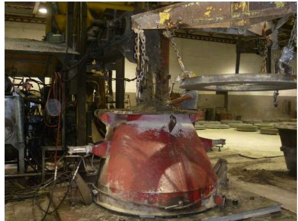
Figure 1. Drycast operator controlling the pouring of concrete into the top cone form mold on the drycast vibration table. Photo by NIOSH.
