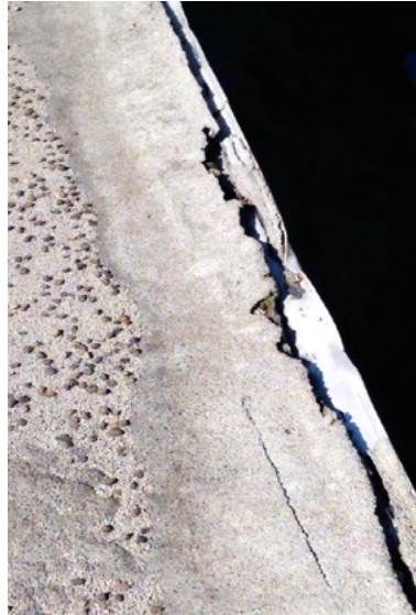
Figure 5. A gap identified at the roof and wall joints of the storage building located near the corn processing area, September 2014.
