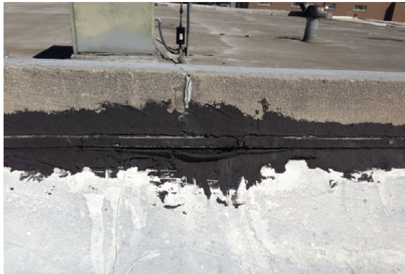
Figure 7. Damaged roof flashing and caulking at the joint between the two buildings of the maintenance department and repacking areas, September 2014.
