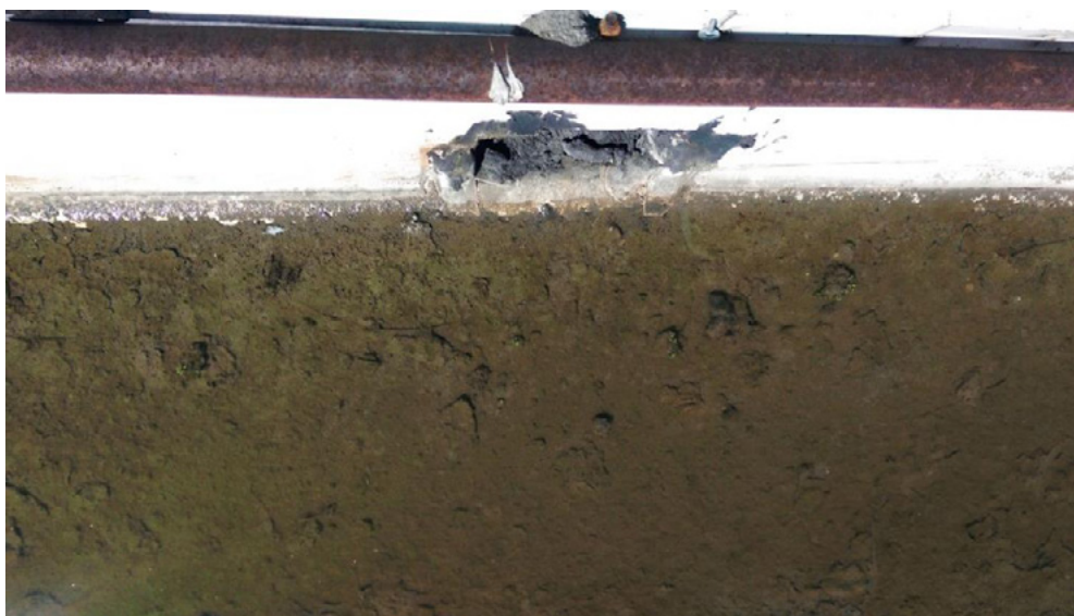
Figure 3. Hole in damaged roofing materials, September 2014. Hole was located near the water pool seen in Figure 2.
