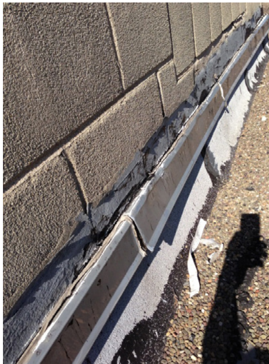
Figure 6. Damaged roof flashing and disintegrated caulking on the roof above the accounting and general office areas, September 2014.
