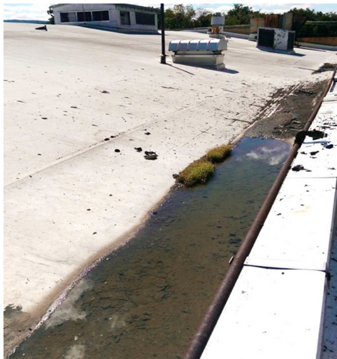
Figure 2. Pooled water near the edge of the gable roof of the chip processing and storage building, September 2014.
