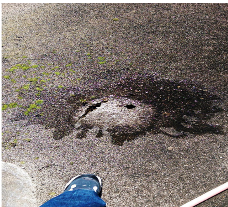
Figure 4. Rain water trapped between two layers of patched roofing materials, September 2014.
