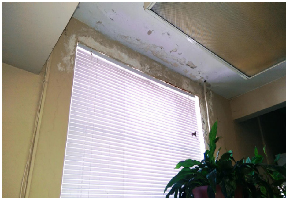
Figure 8. Water intrusion near an office window, September 2014.
