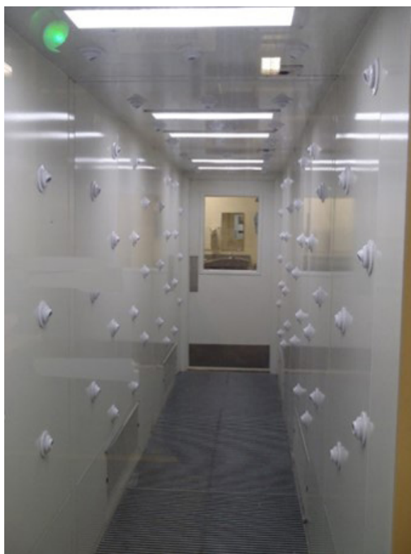
Figure 5. Air shower tunnel viewed from production area into nonproduction area hallway. Photo by NIOSH.
